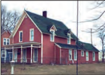
223 State Street; 3 apartment units; work in progress 1 unit nicely done
