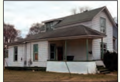
419 State Street; 2 apartment units
